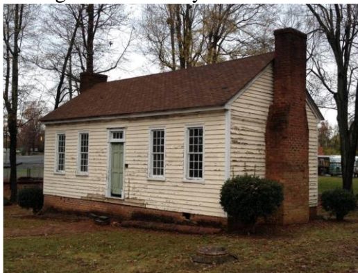
The 1976 restoration after a period of deterioration.
