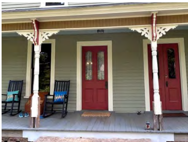
Victorian adornments: top — pre-1890s gable end with vent; post-1890s gable end with window and Eastlake-style bargeboards. Middle — gable end; cornice bracket detail. Bottom — front porch detail with corbels and brackets and turned posts; bracket detail.
