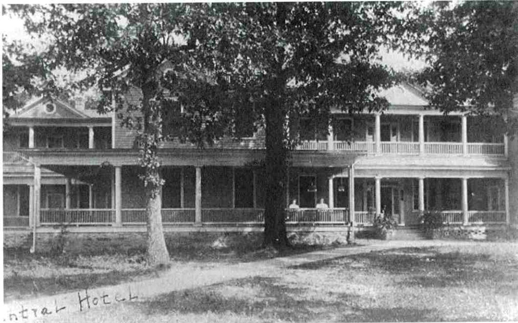
Central Hotel, west elevation, 1910
