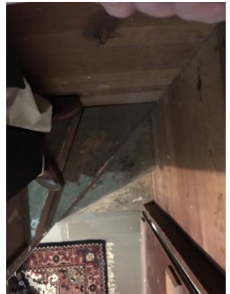
Staircase detail—top view
