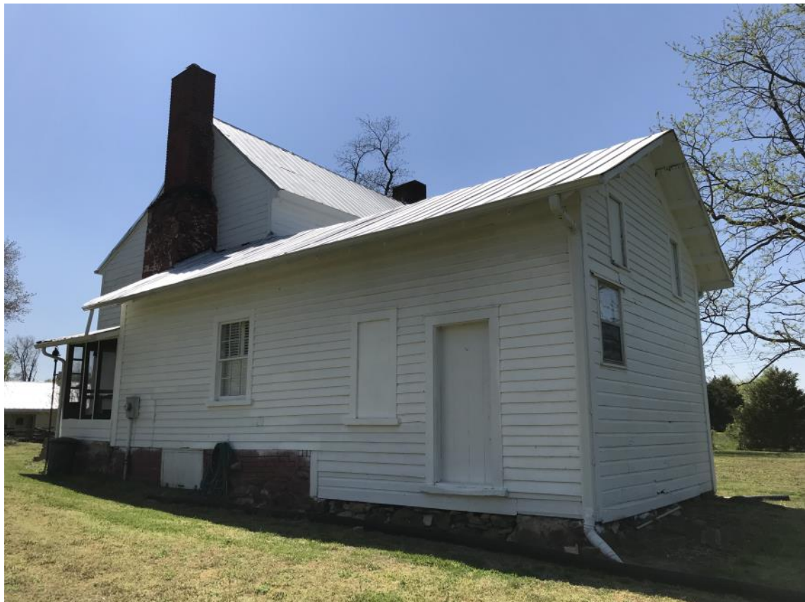
Rear view from northeast with kitchen wing
