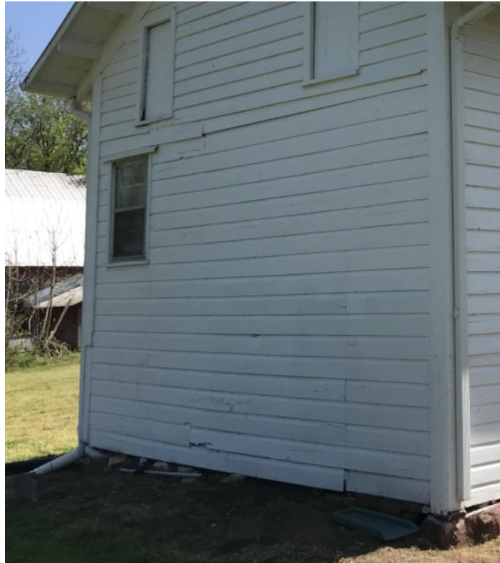
Location of kitchen chimney
