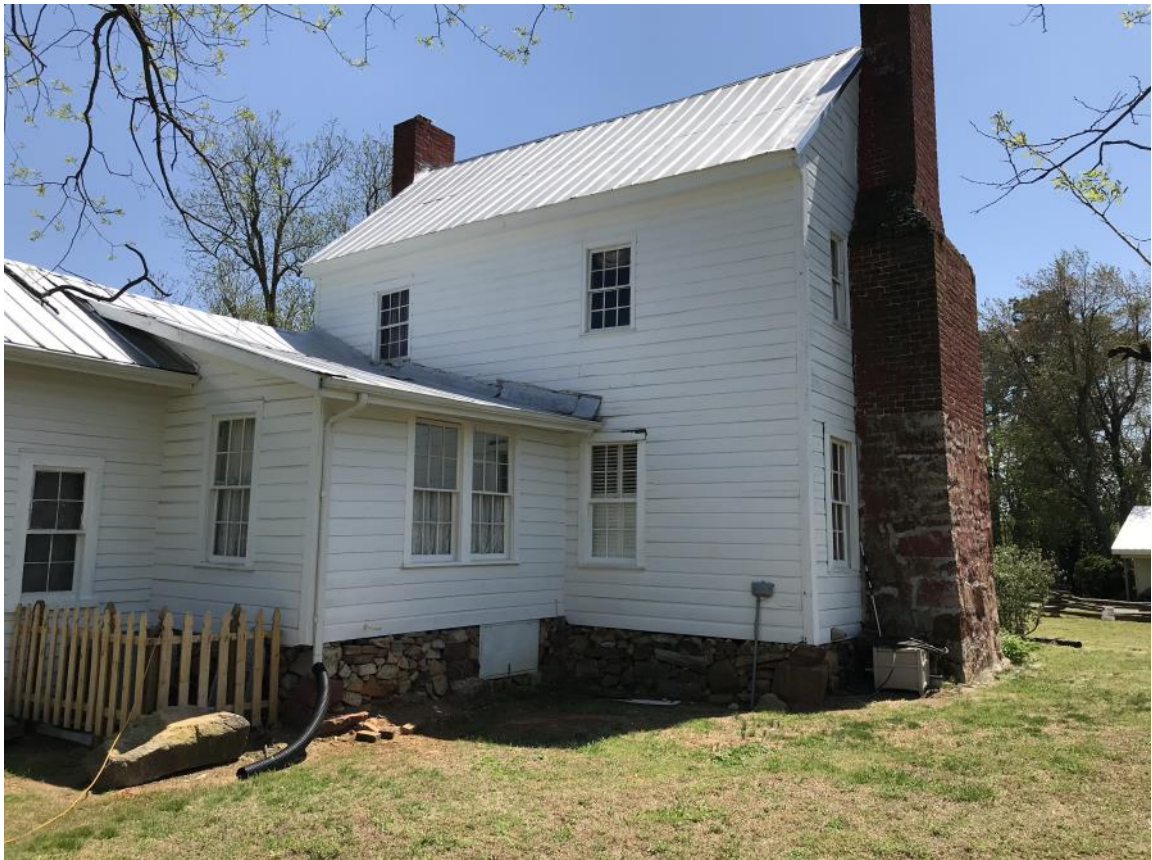
Rear view from northwest
