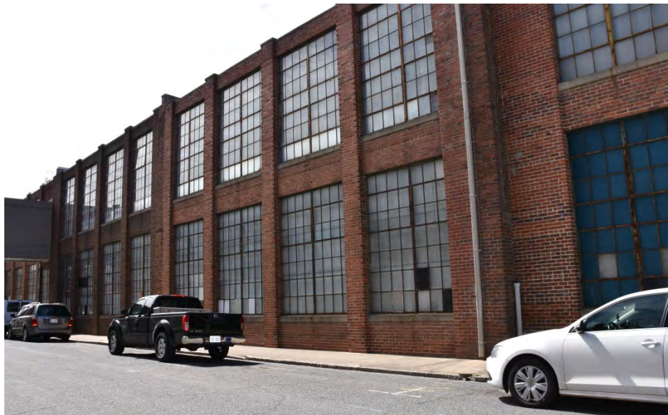
1924 (top), 1928 (center), and 1929 (bottom) additions, east elevations
