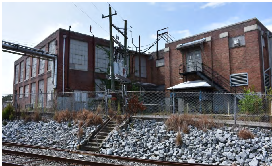
Southwest oblique (top), east elevation (center), looking southwest (bottom)
