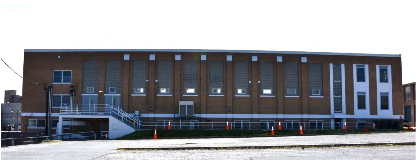
Southwest oblique (top), southeast oblique (center), and north elevation (bottom)
