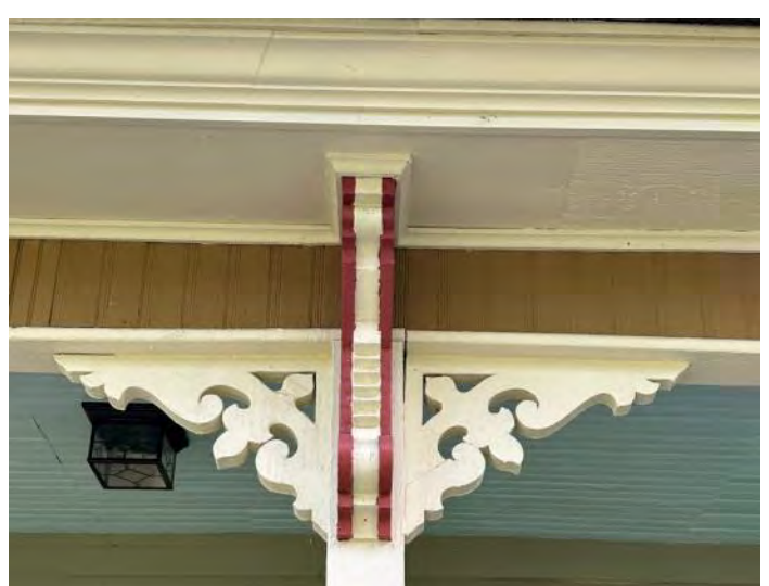
Victorian adornments: top — pre-1890s gable end with vent; post-1890s gable end with window and Eastlake-style bargeboards. Middle — gable end; cornice bracket detail. Bottom — front porch detail with corbels and brackets and turned posts; bracket detail.
