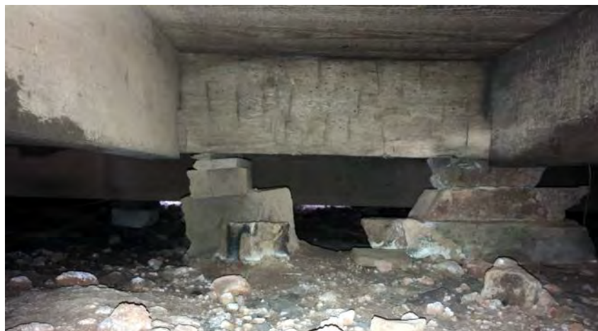
Top — Pre-1890 prior to addition to northern end; middle — house in 1979; bottom — hand-hewn beams under central portion of house
