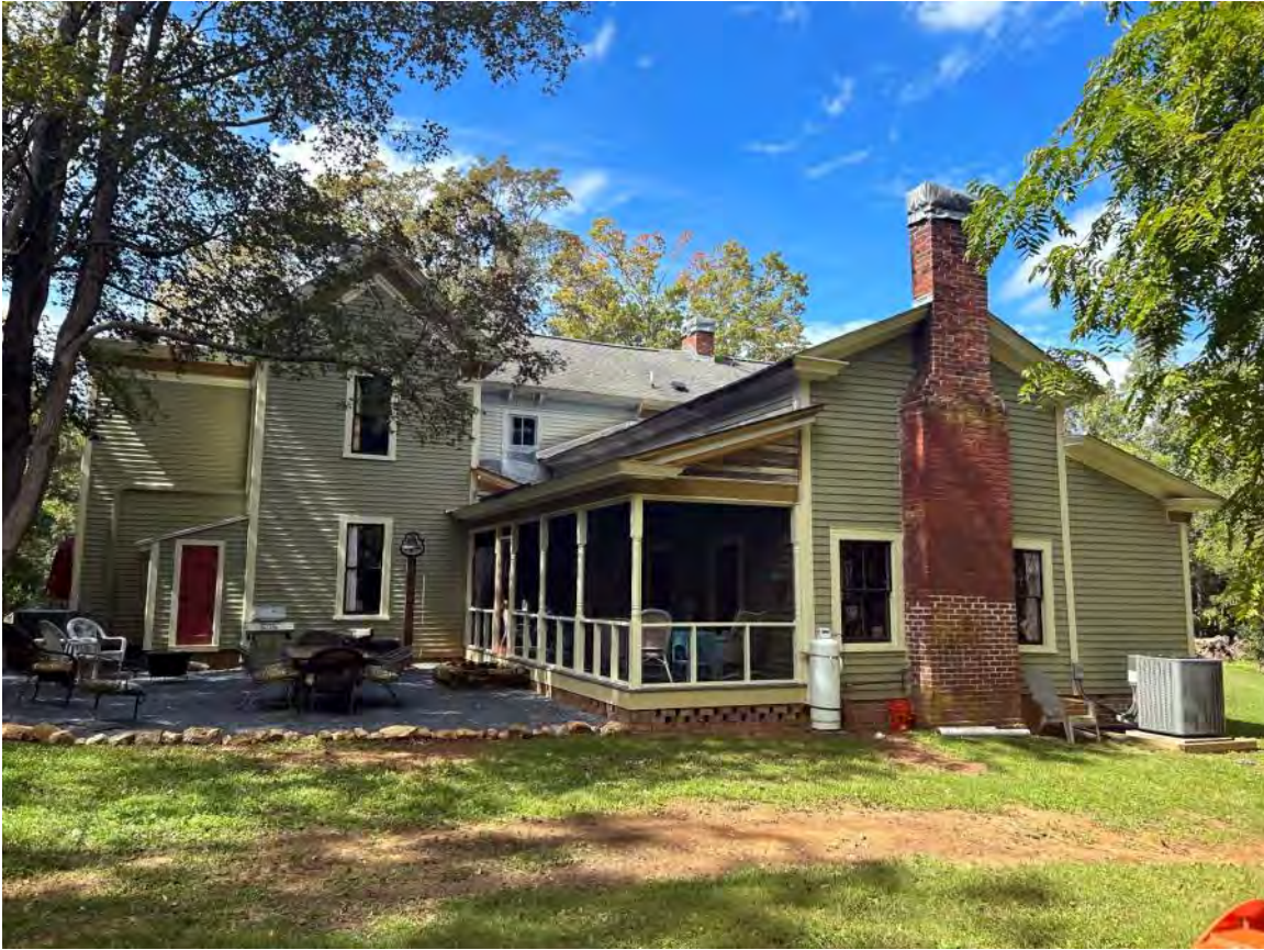
East elevation, top showing ell created by enclosures of formerly detached kitchen; north elevation showing north side of ell, bottom
