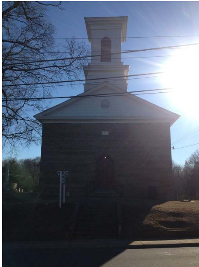
Figure 4: St Paul's Church; front view from High Point Street
