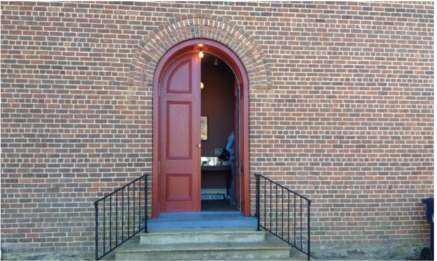
Figure 3: St Paul's Church front door
