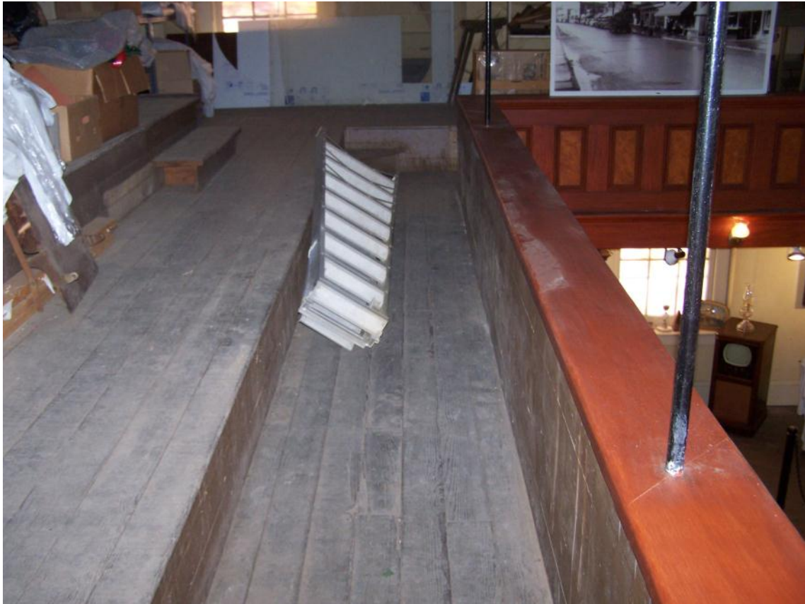
Wide plank flooring in balcony
