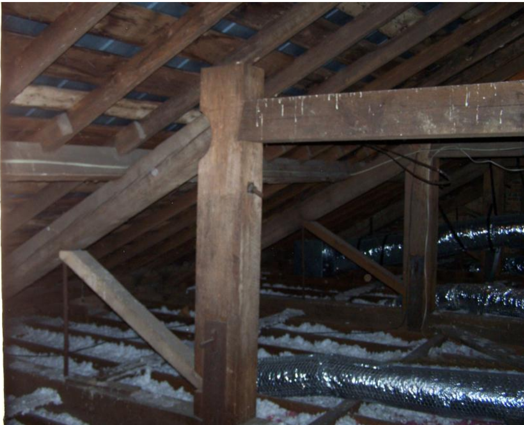
Original wood beams in attic area
